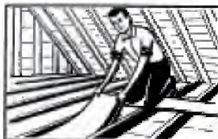
Tells how to install Gold Bond Rock Wool Blankets between joists of unhoored attic.
